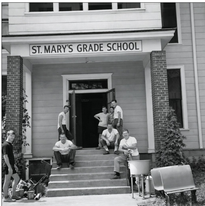
Cleaning out the St. Benedict's Academy / St. Mary's grade school before demolition.
